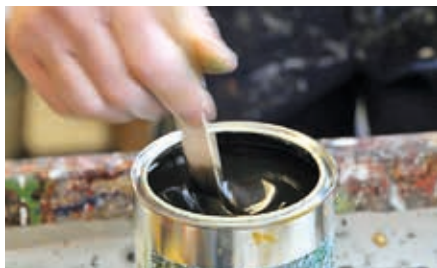
Stir the paint thoroughly before painting.
