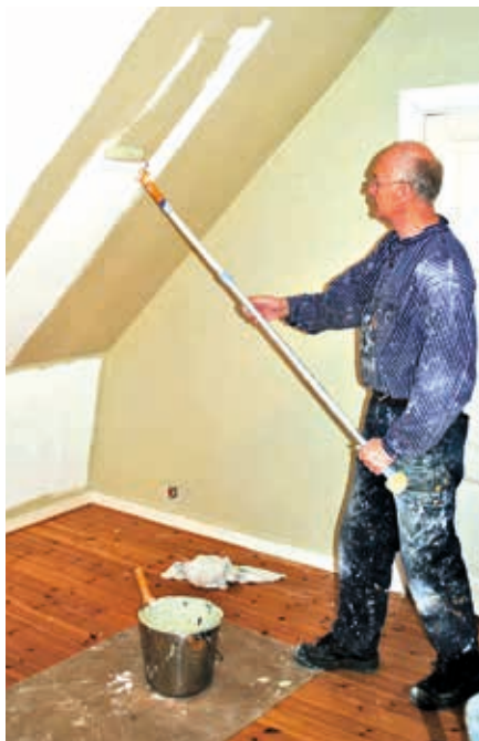
Painting papered walls with a roller.
